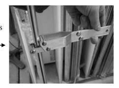
Hold the Guide Arm attached to the Guide Poll up to the top corner of the window. The top of the Guide Arm should be resting 25mm in and 25mm up from the bottom edge of the Hood Box. While holding the Guide Arm in this position, mark the holes for the Guide Pole hanging from the Guide Arm.
