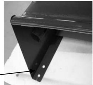
Screw in either hole that is not on a mortar line
