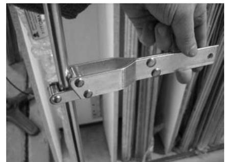
Hold the Guide Arm attached to the Guide Poll up to the top corner of the window. The top of the Guide Arm should be resting 25mm in and 25mm up from the bottom edge of the Hood Box. While holding the Guide Arm in this position, mark the holes for the Guide Pole hanging from the Guide Arm.
